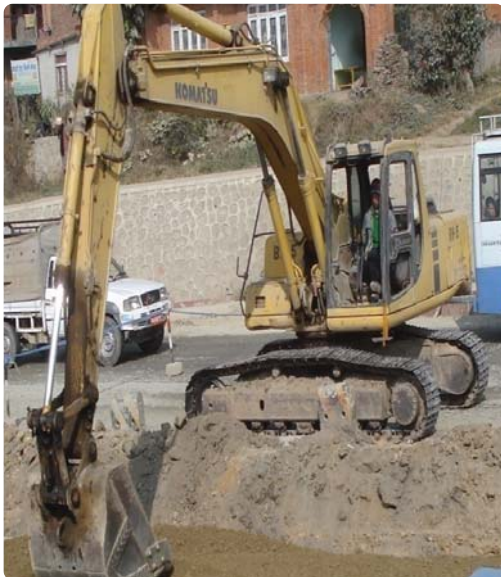
Excavator at work
