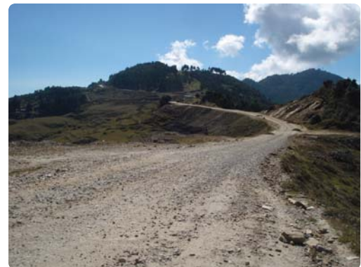
A ridge alignment in Dolakha that may be ideal for EB technology to expedite road construction
