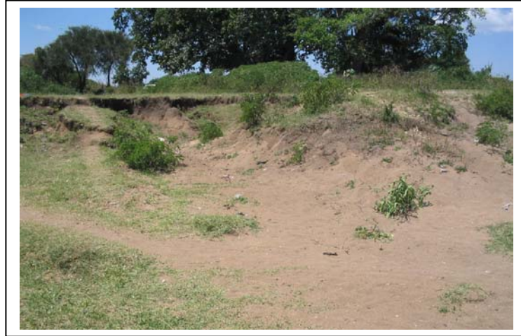
Figure 5: Erosion due to sand harvesting at Kamariga Beach (Picture), the raised part is a public path
