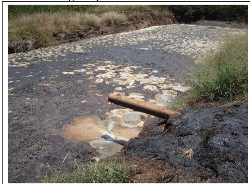
Figure 4: 1 st aeration pond of Bondo Fishmeal Ltd, the white layer is murky fat that does not allow air and sunlight to penetrate to assist in treatment
