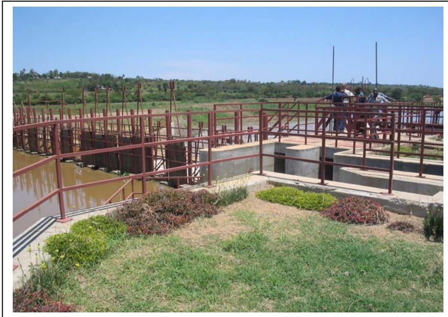
Figure 2: Dominion Farms river weir
